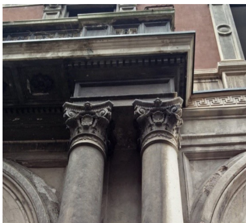
Figure 1. Example of black crust formation.
