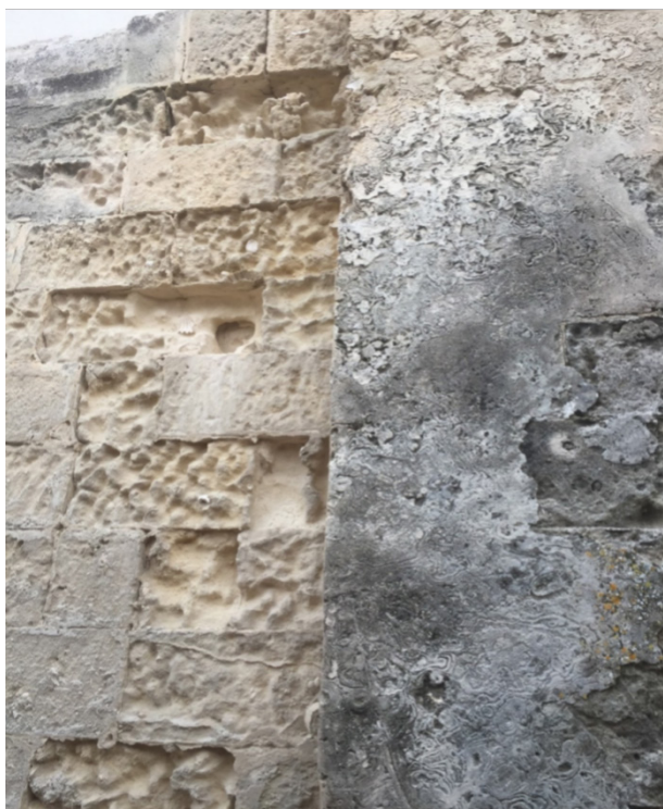
Figure 2. Detail of a masonry with varying degrees of alveolization of contiguous ashlar.
