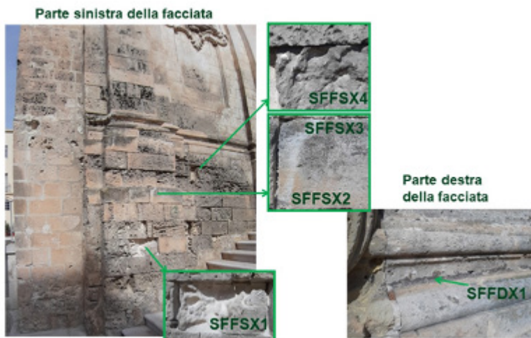
Figure 7. Sampling of the front façade of San Francesco d'Assisi.
